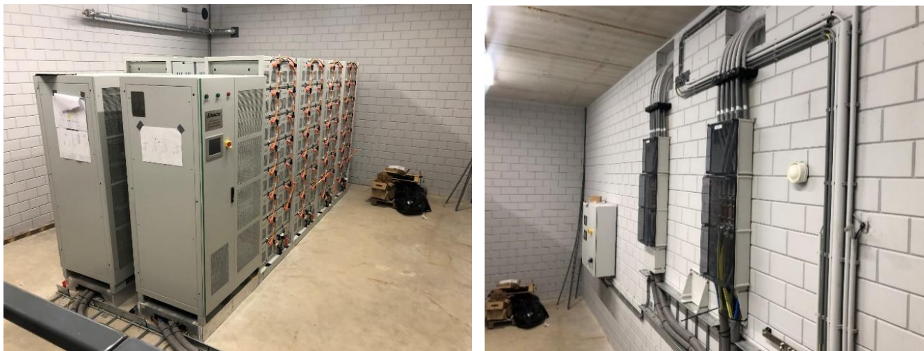
Figure 3-10 Li-ion battery installed
