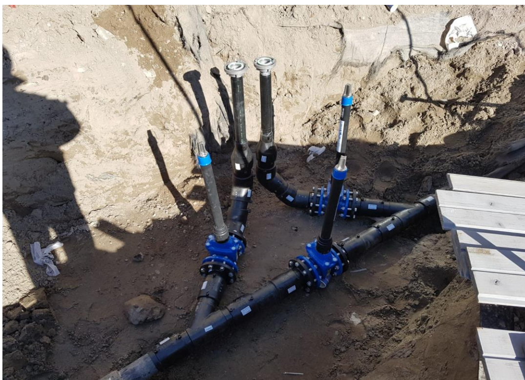
Figure 7-3 Underground piping of the vacuum system
