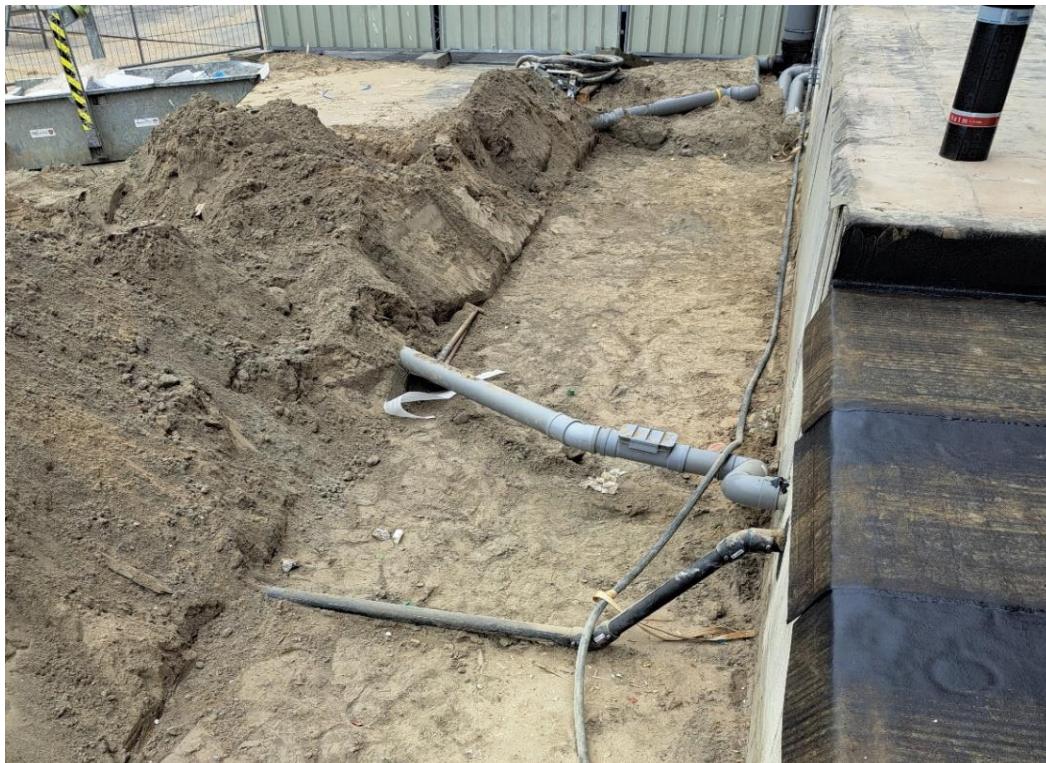
Figure 7-4 Connection to the vacuum sewage on the Republica side.
